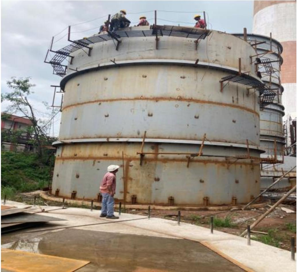
A photograph of a large cylindrical process water tank under construction. The tank is made of light-colored metal with visible rust. Workers are on top of the tank, and scaffolding is visible around it. A worker in a pink shirt and white hard hat stands in the foreground near a concrete base. |
