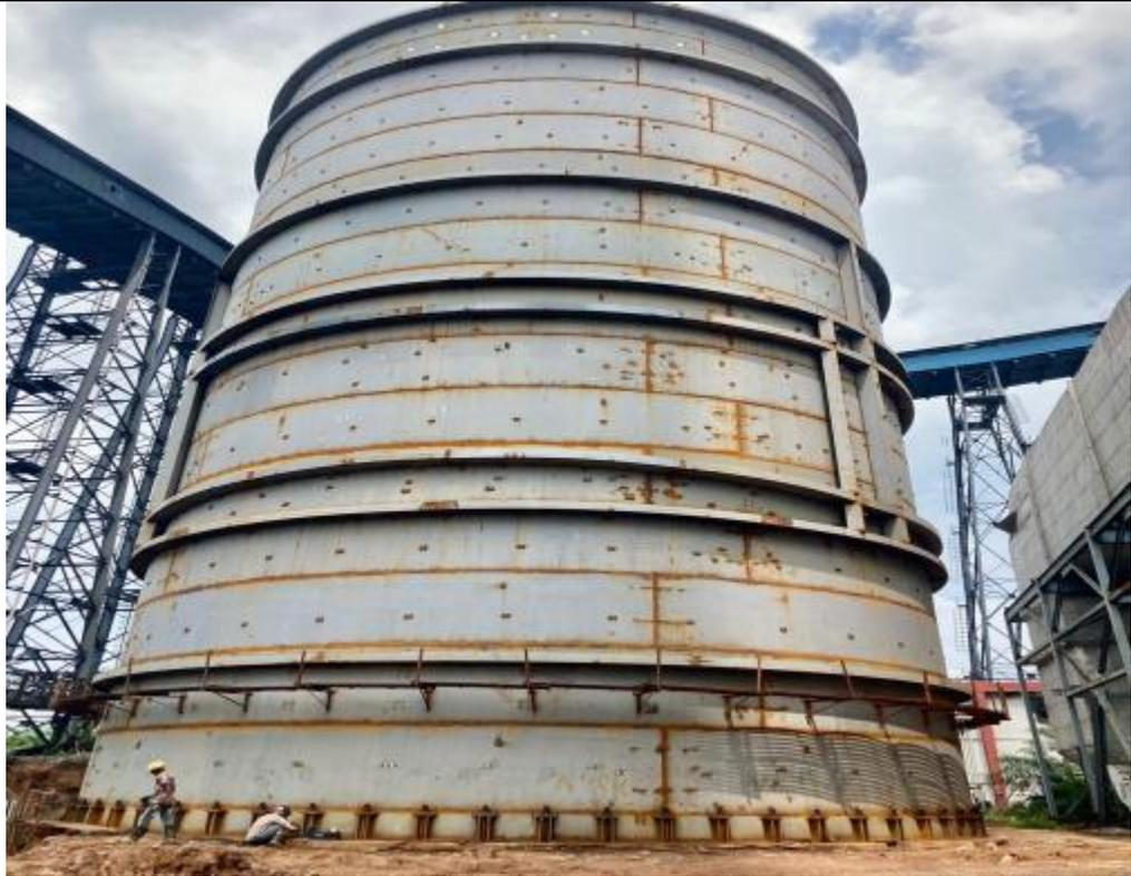
A large, cylindrical industrial absorber tank, labeled Absorber-2, is shown under construction. The tank is composed of several horizontal sections of galvanized steel, showing signs of rust. It is situated outdoors at a construction site, with a blue steel structure and other industrial buildings visible in the background. Two workers are visible at the base of the tank. |
