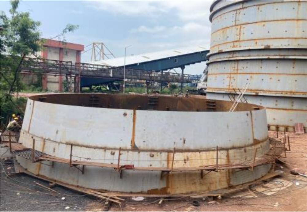
A photograph showing a large, cylindrical, conical portion of a tank under construction. The structure is made of light-colored metal panels with visible rust and is supported by a wooden platform. In the background, there are other industrial structures, including a tall cylindrical tank and a building with a red roof.             |
