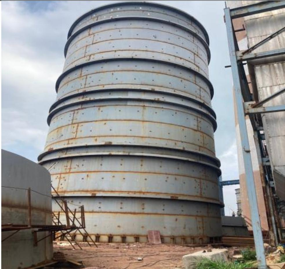
A large, cylindrical industrial absorber tank, labeled Absorber-1, is shown under construction. The tank is composed of several horizontal sections of galvanized steel, showing signs of rust. It is situated outdoors at a construction site, with a blue steel structure and other industrial buildings visible in the background.                                                 |
