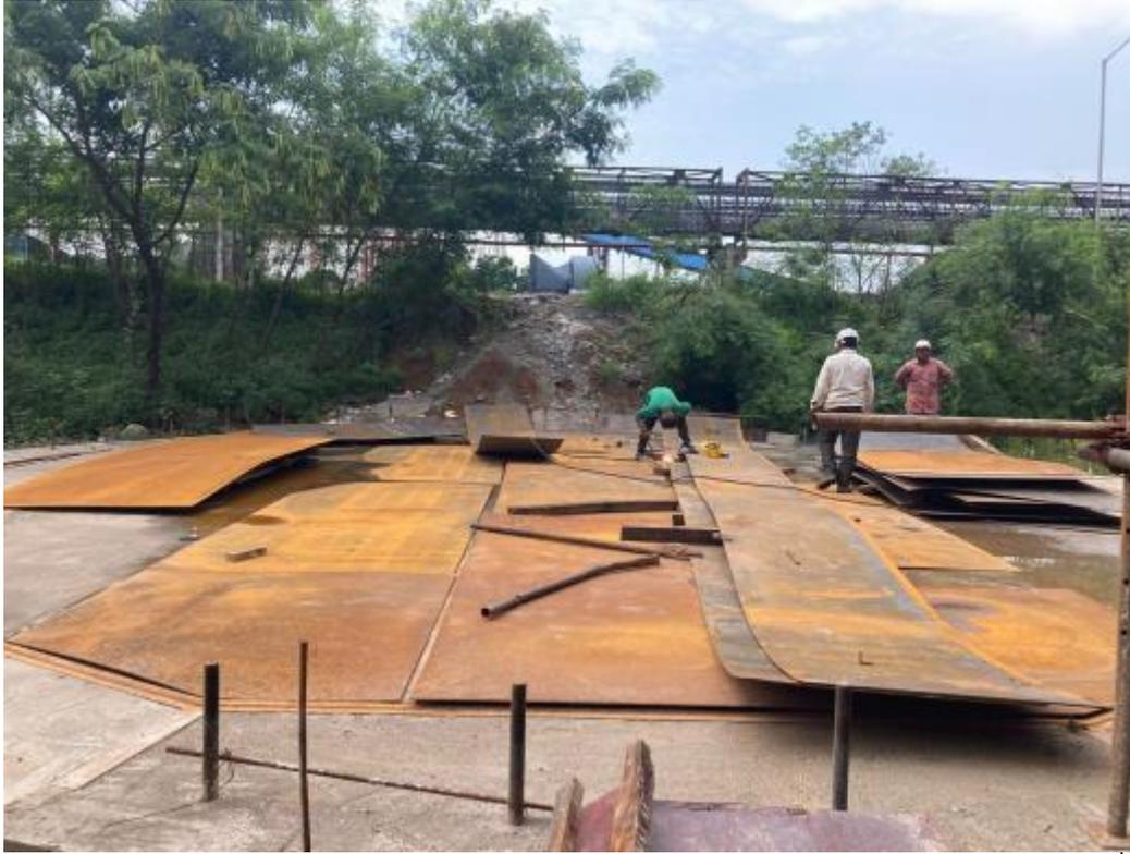
A photograph showing the construction site for an emergency storage water tank. Large, rusted metal plates are laid out on a concrete base. Several workers in hard hats are visible, some standing and some working on the plates. The background shows trees and a building.                           |
